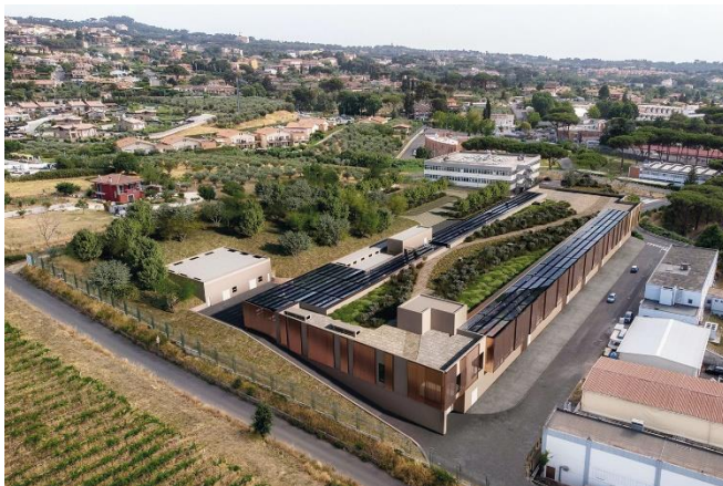
Image 1: Projected building for the particle-driven plasma accelerator of EuPRAXIA in Frascati, near Rome. © INFN & Mythos - consorzio stabile s.c.a.r.l., Italy.
